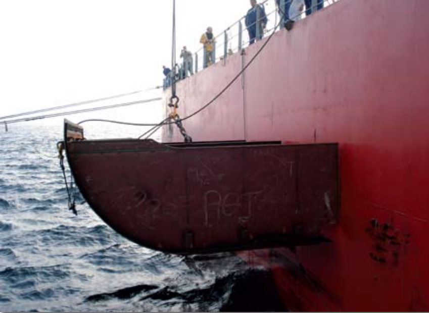
The new prefabricated section being lowered into position to be inserted into the (5 x 5mtr) cut-out in the hull using chain blocks.
